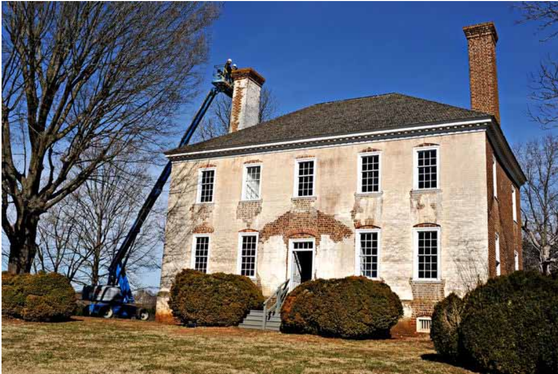
Tony Beal, a structural engineer, and Jimmy Price, a brick-and-mortar specialist, inspect the chimney of Salubria in Culpeper for a report on needed preservation work.
